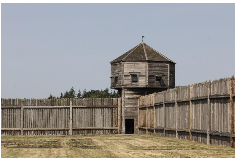
3 - The 1845 corner bastion at Fort Vancouver, a U.S. National Historic Site along the Columbia River in Vancouver, Washington
